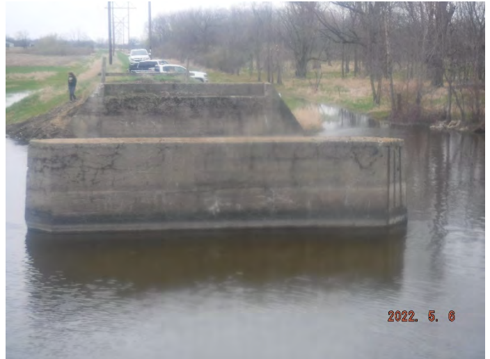
East Face of Pier
