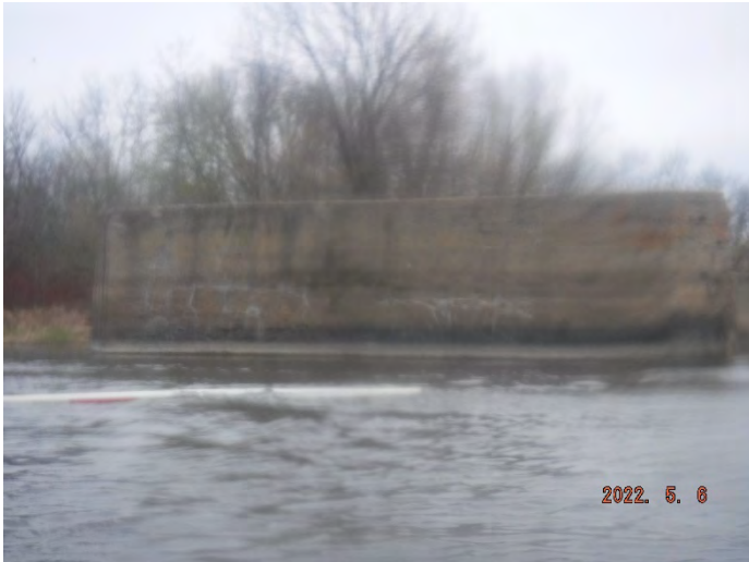
West Face of Pier
